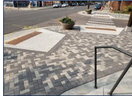
Figure 4. Existing Pedestrian Ramps
